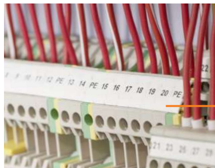
DEK/WS/MF: Flexible connector markers - print, clip, finished
